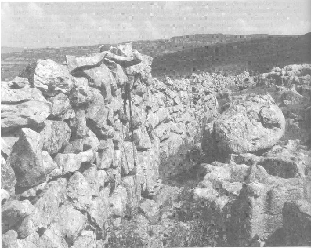
Figure 18.6. Wide top double wall with projecting topstones built on limestone pavement near Darnbrook.
