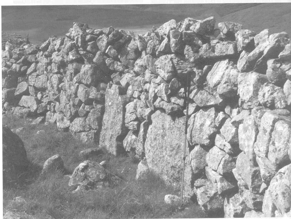
Figure 18.5. Orthostats at the base of a wide top double wall near Darnbrook. The original topstones are missing.
